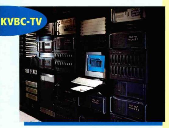
Profile video server room. A combination of Profile PDR400s, with native DVCPRO format recording and the PDR200s for on-air clips make a powerful team for the stations' fast-pace news operation. Two ingest PDR400s provide 22 hours storage each. Material to be edited is transferred to PDR200s over Fiber Channel.
