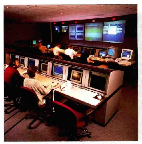
Illuminet's Network Surveillance Control Center, Overland Park, KS. Control centers such as this monitor a network of public-switched telecommunications infrastructure, helping to ensure an even spread of traffic and the highest access speeds available. Photo courtesy Illuminet.
